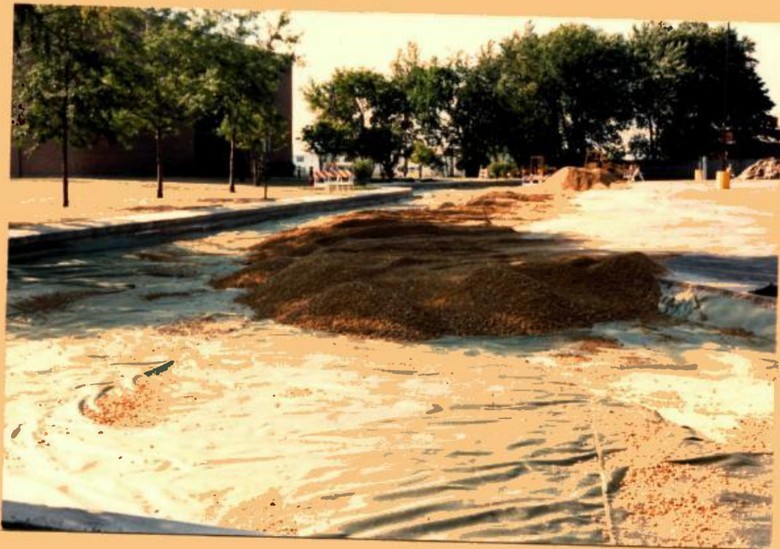
INDIAN TRAILS PUBLIC LIBRARY PARKING LOT CONSTRUCTION- 1987
